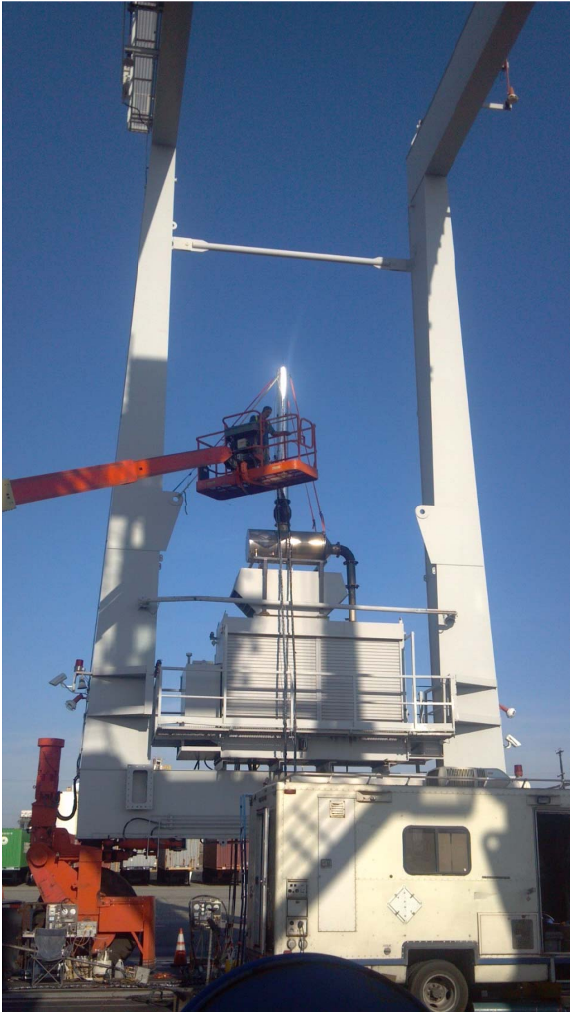
Photo 2: Best Environmental team conducting emission measurements
